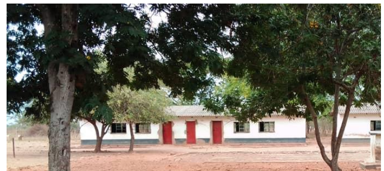
Hwata Secondary –July 2022, after repairs
